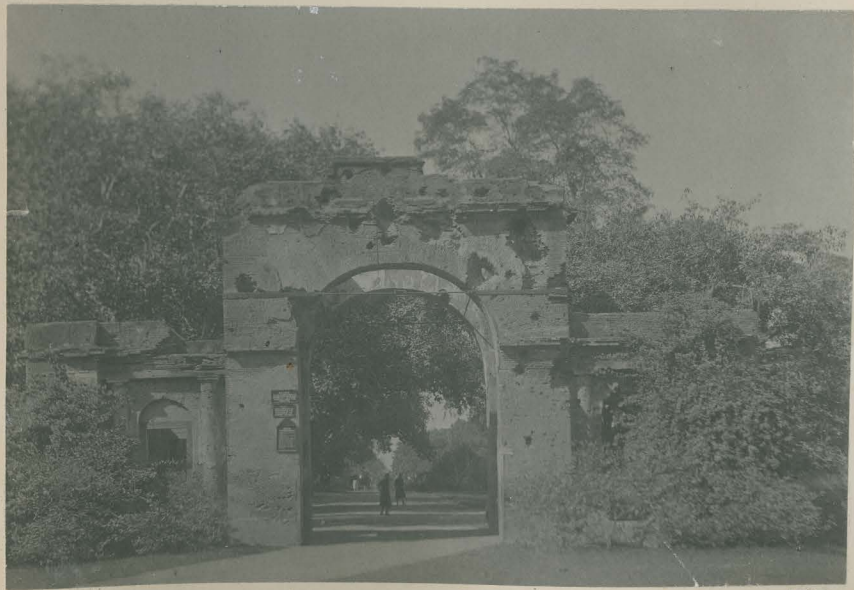
E. Bailey Guard Gate Lucknow - commanded by St. Aithens the 13 th N.Y. on entering of Asper House is on the left - the banqueting hall on the right. here did Sir H. Lawrence. In a room here the Enfield cartridges were made from Jewell's mould.
